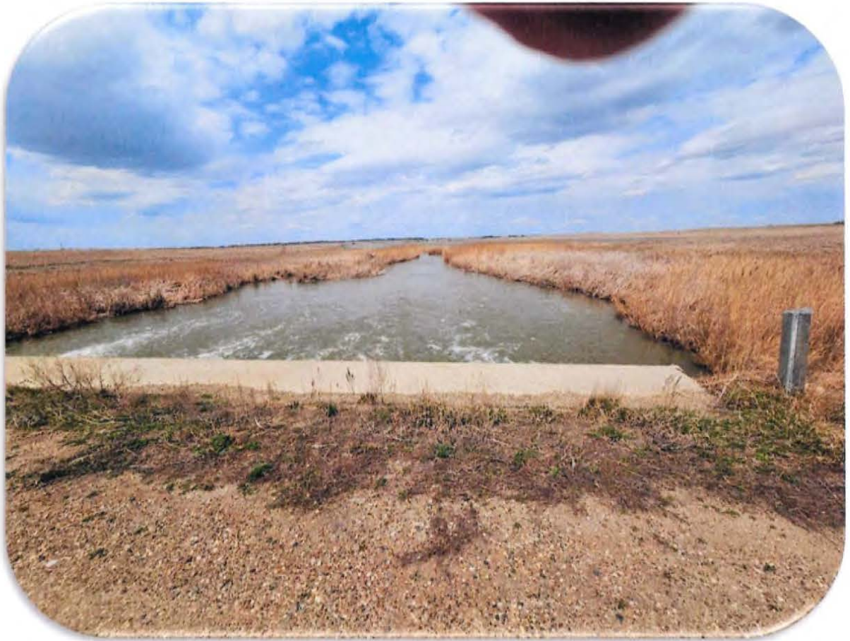
Looking North downstream from the LLR spillway toward Hwy #83
